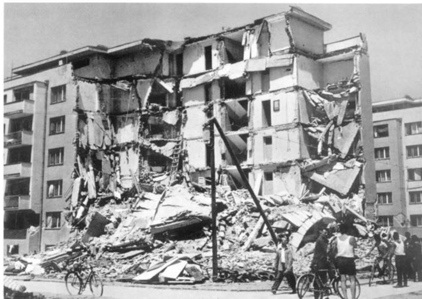
Fig. 5. Failure of right side structural unit of five story apartment masonry building in the West side
